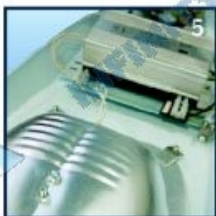
Adjust the clips to tightly secure the fixture and fasten with butterfly nut
