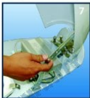
Completed ballast connection
