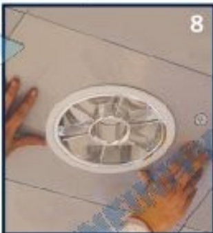
Install the fixture and tile into dropped ceiling
